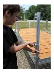
5. The existing dock leg is already aligned with the inner dock frame so the second double socket will mount with the open socket beside the pipe.
