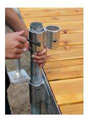
4. Attach a double socket to the top of this pipe with one side over the decking.
