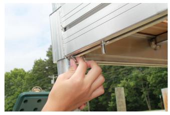
1. Slide two carriage bolts down the bottom track to receive the pipe bracket.
