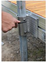
3. If the pipe bracket is in the correct position for your bench, drive a pipe through the pipe bracket into the ground then tighten the set screws and nylock nuts.
