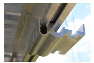
3. The small ridge on the back side will make a click noise when it secures to the grove on the under side of the dock frame.
