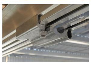
4. The Section being added will rest on the J-Brackets and each J-Bracket will receive a carriage bolt and nut in one of the two slotted holes in The J-Bracket.
